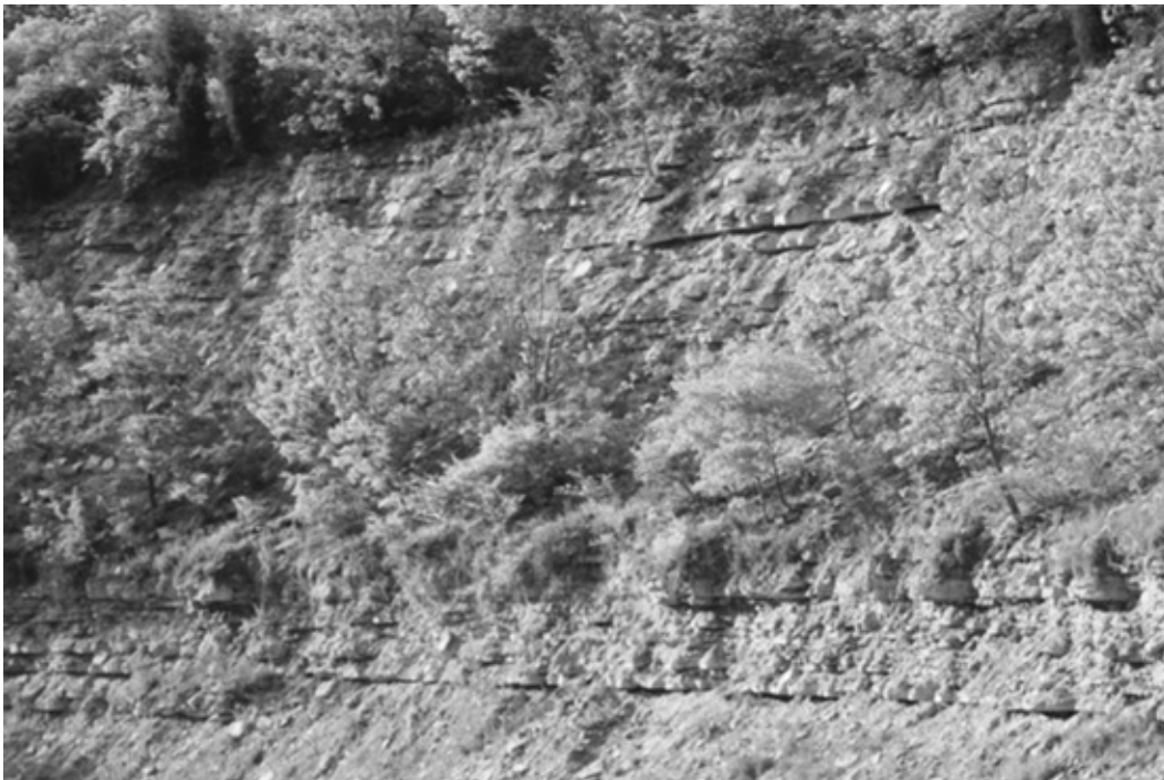
Figure 5. Alternating beds of limestone (hard) and shale (soft) in the Fairview Formation in a road cut in the Cincinnati area of northern Kentucky. (Photograph: Andrew A. Snelling)
