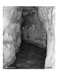
The tunnel ranges in height from  $5\frac{1}{2}$  feet to as high as 16 feet. It runs 1,748 feet long. The tunnel is almost level, dropping only 12.5 inches in the course of its total length. At its deepest, it is 150 feet below the earth.
